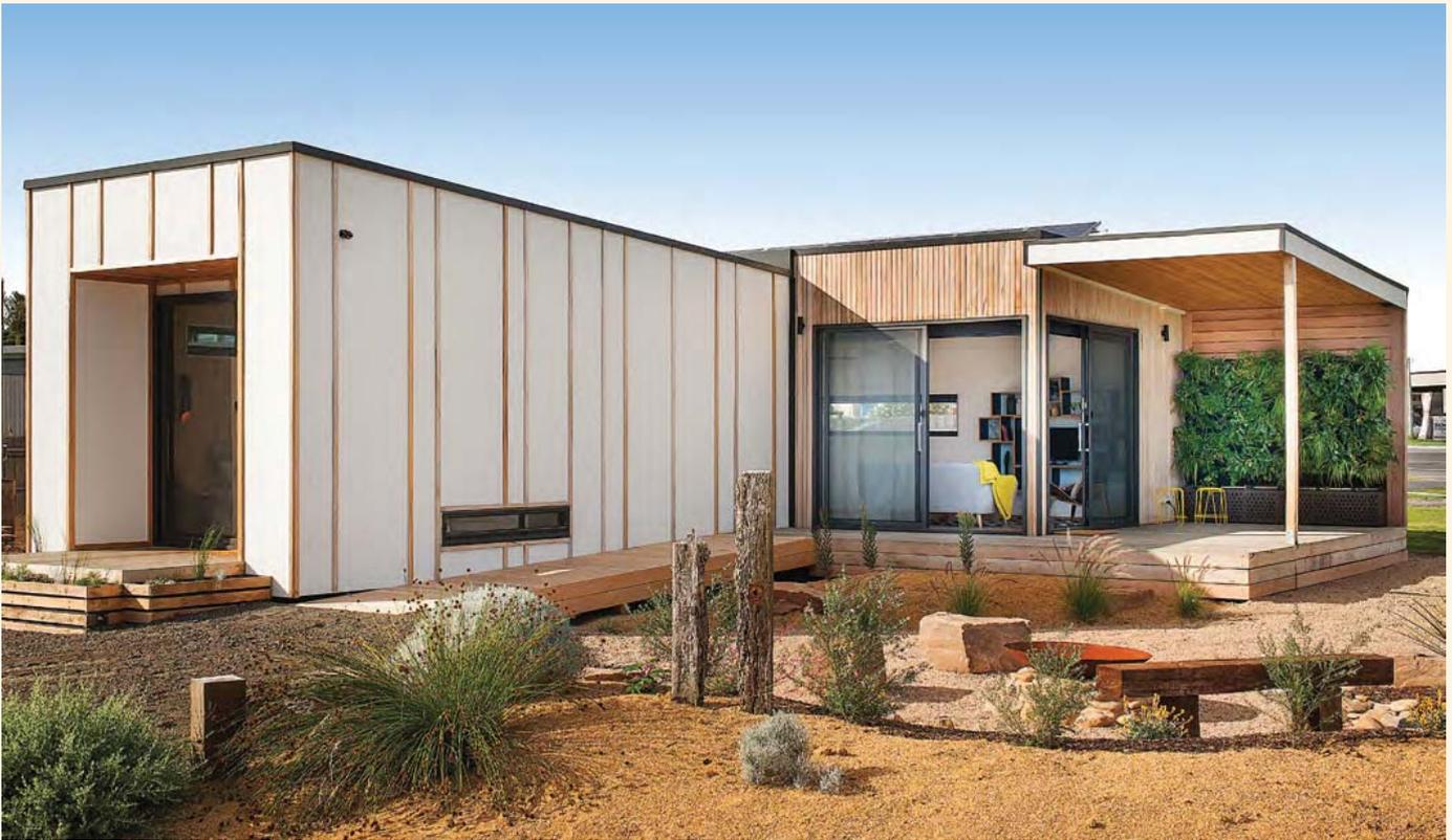
Material selections for the prototype modular dwelling were selected for low embodied energy and low toxicity. Weathertex and Radial timber cladding were used for the exterior and BlueScope steel for the roof. Image by Warren Reed.
